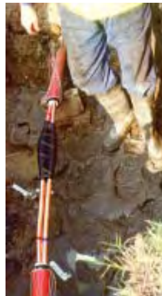
SOJ 12 kV on a cable with copper tape screen, China.
