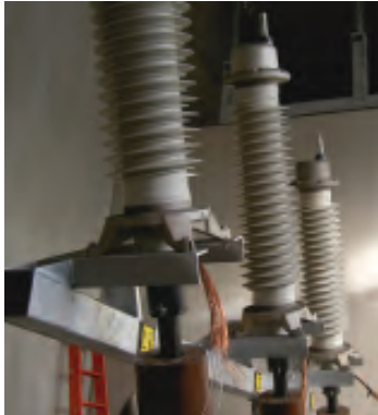
APECB-P 145 kV with composite insulator, Sweden.
