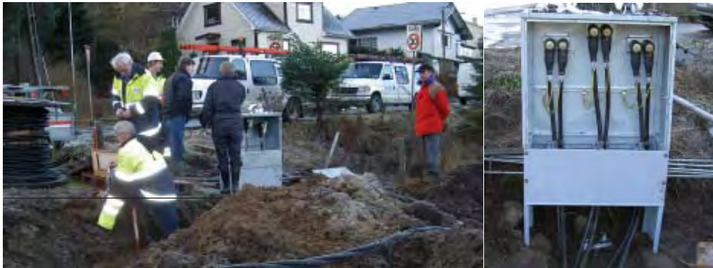
Installation of HDC 630 at Farsund, Norway.
