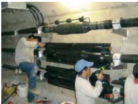
Assembling premoulded cable joints, SMPGB-C.
