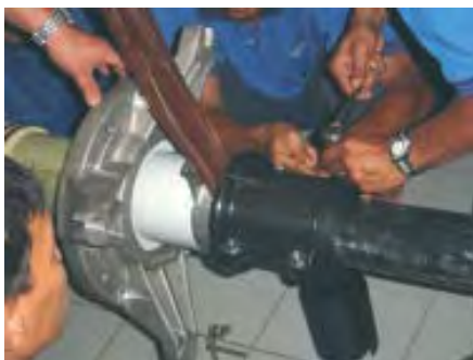
Our cable terminations can be mounted with care horizontally on the ground and then lifted into place, both easily and safely!
