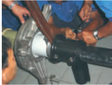
APECB 145 kV with porcelain insulator, high voltage training, Malaysia.
