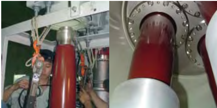
APEGA 170 kV at GIS (gas-insulated switchgear), Taiwan.
