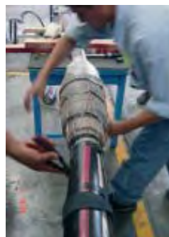
Assembly of premoulded cable joint JS.
