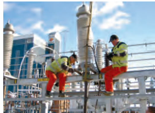
APECB-P 145 kV with composite insulator, Sweden.
