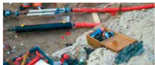
Transition joints SMTXB 12 kV, The Netherlands.
