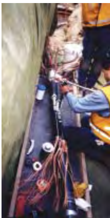
SOJ 24 kV, with screw technique, Australia.
