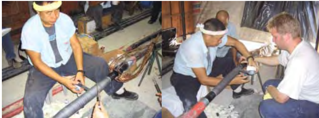
SMX 72 kV which supply a casino at Macaus harbour in China with electricity.
