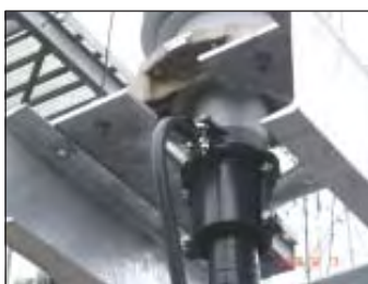
Base part and cable clamp.
