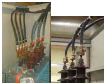
SOT 12 kV at transformer, Sweden.
