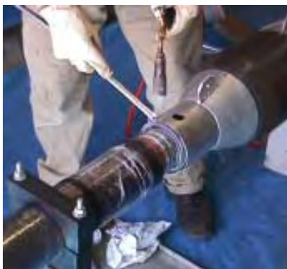
Installation tool, RKM 170 for mounting SMPGB on a 170 kV cable.
