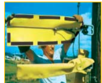
Installing a Zip-On Blanket
