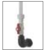
Sight Glass with single isolation valve
